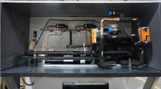
Figure 12: PR Water Coils Configuration
